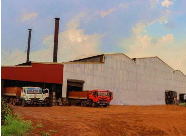
Unit-IV: Green-Field No-Brake Foundry Shed & Shop-Floor
